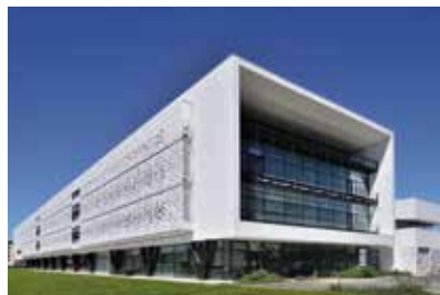
INSTITUT D' OPTIQUE D' AQUITAINE Location: Talence, France Studio: Cabinet d' architectes Nicolas Raguenau & Antonie Roux
