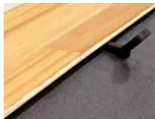
3. Press Into Place Presionar Compression
