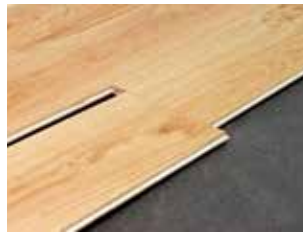
3. Press Into Place Presionar Compression
