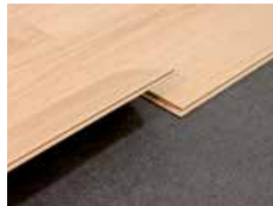
2. Press Into Place Presionar Compression
