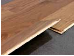
2. Press Into Place Presionar Compression
