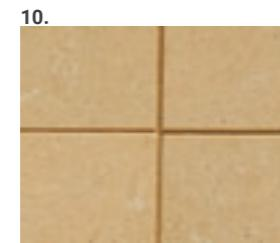
9/ Before grouting the tiles, make sure that the tile joints are clean and free from any bonding material or dirt. This type of substance can detract from the end result of the tile joints and also reduce the bonding strength of the grout.
