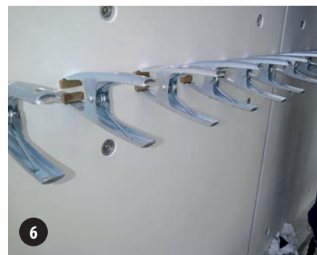
The fastening clips are installed so they exert pressure and ensure a perfect joining of the two slabs.
