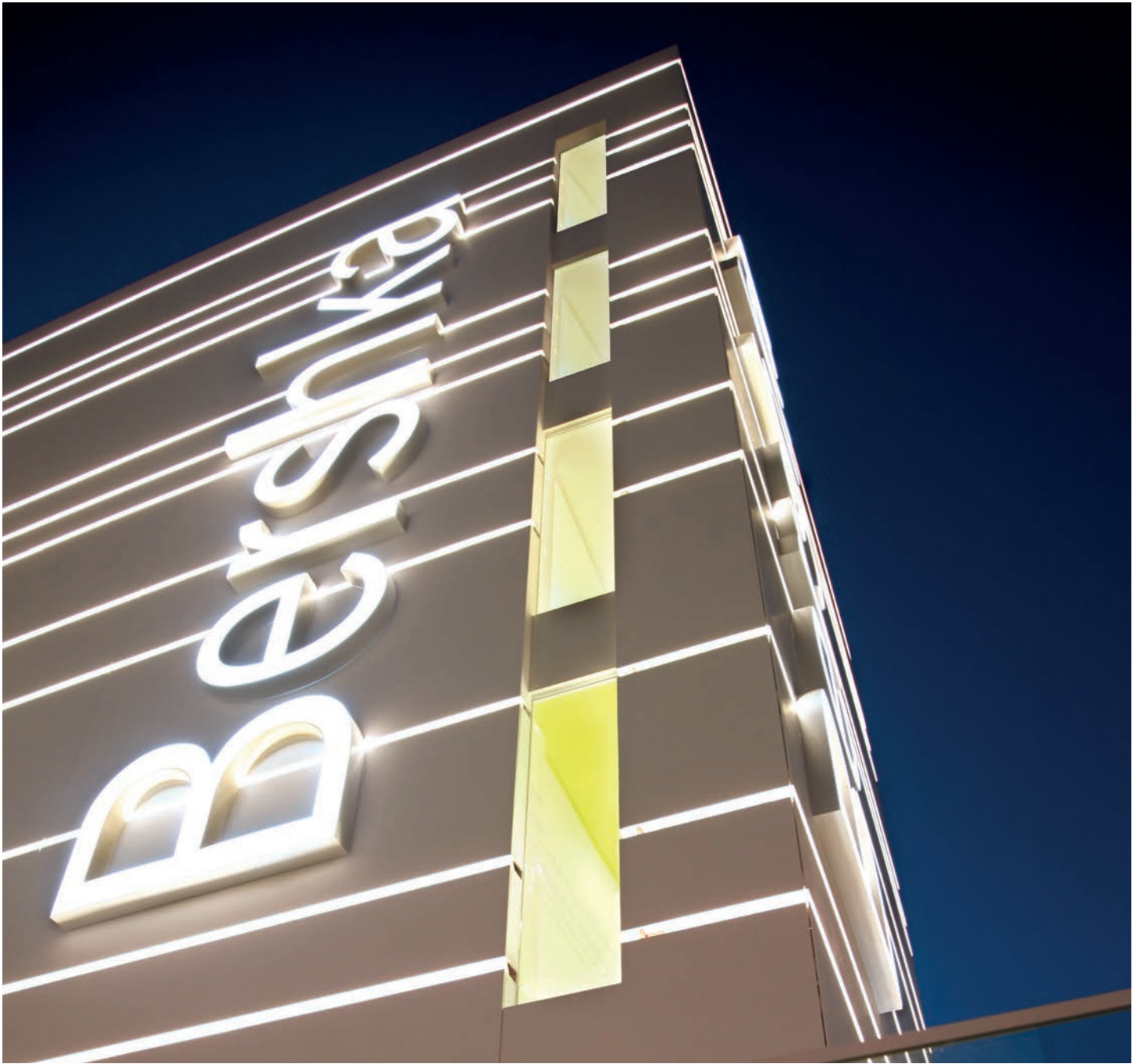
Bershka shop in Istanbul, Turkey. Architects: Castelvejana Arquitectura.
