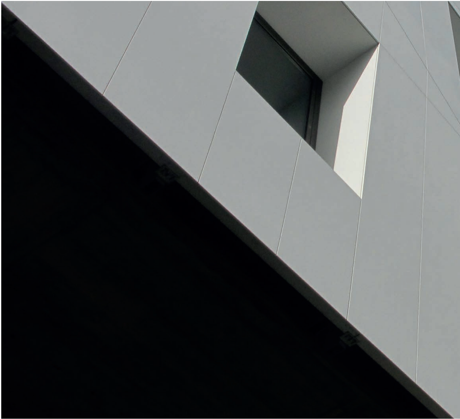
Tour Raffinity building in Casablanca, Morocco.
